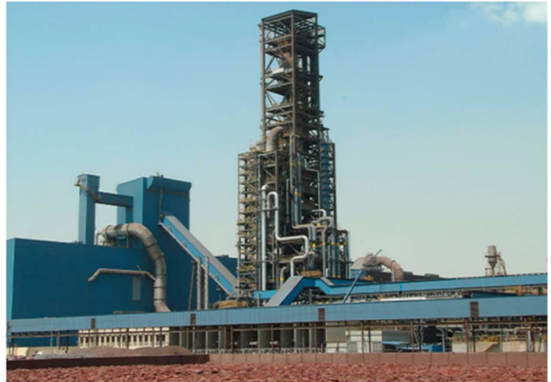
An example of a MIDREX direct reduction plant
