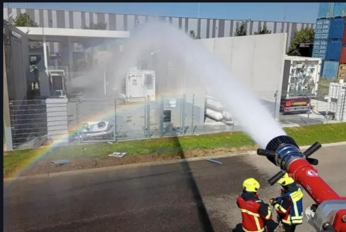
The local fire brigade pouring water onto the source of the fire at the hydrogen refuelling station in Gersthofen, Bavaria. (Photo: Gersthofen Fire Brigade)
