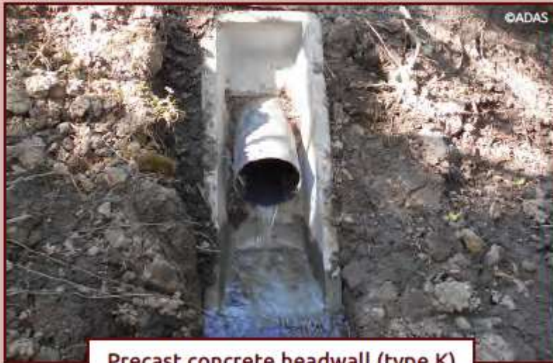
Precast concrete headwall (type K)
